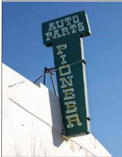
Marquee sign projecting above parapet.
