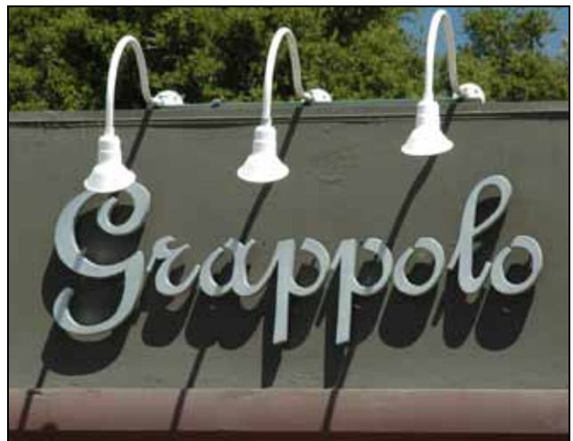
Metal wall sign, offset from building facade.
