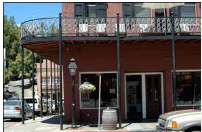
A one-story gallery with second floor access.
