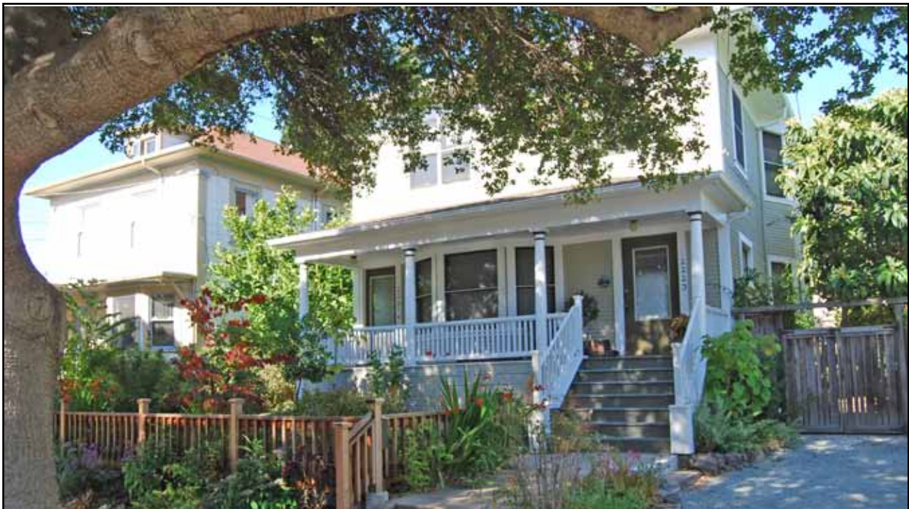
The difference in the form between this duplex and single-unit houses in the neighborhood is barely perceivable.
