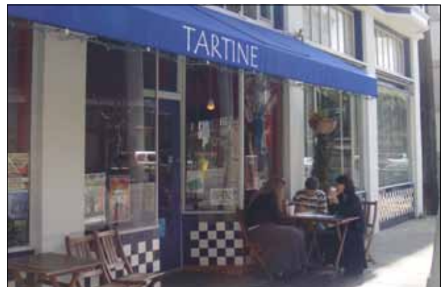
An example of a shopfront with a recessed doorway.
