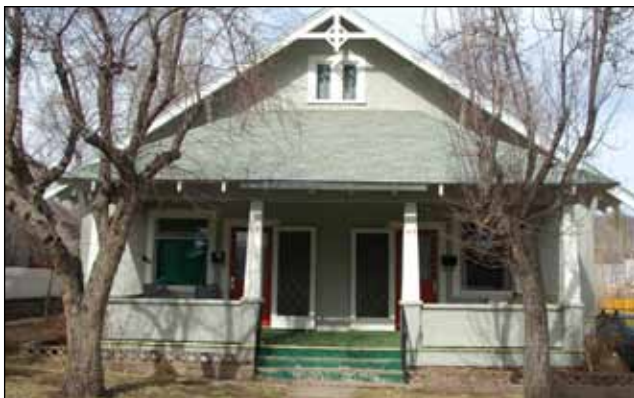
A side-by-side duplex with a shared porch.
