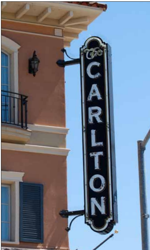
Marquee sign at corner terminating at eave.
