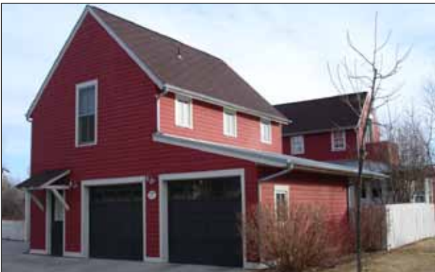
One-and-a-half-story carriage house with an internal stair.
