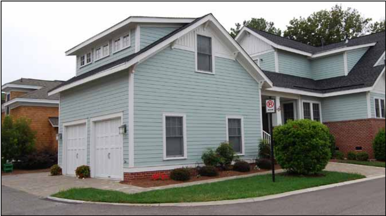
One-and-a-half-story carriage house connected to main house by a breezeway.
