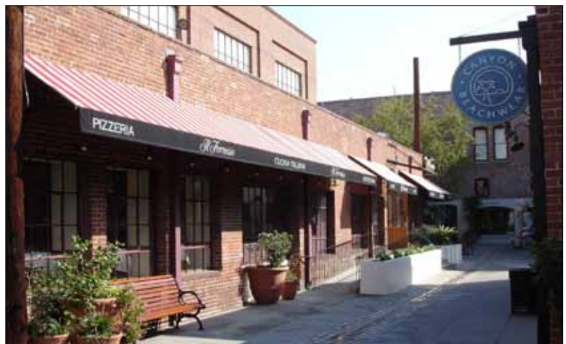
Series of awnings along a frontage.
