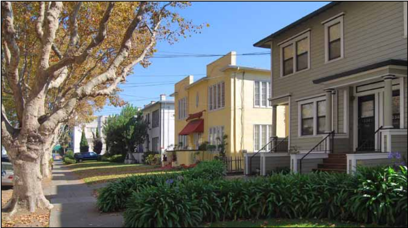
A group of apartment houses that have the scale and character of large single-family houses.
