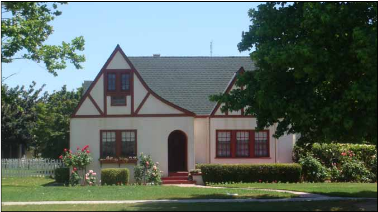
One-and-a-half-story front-loaded village house.
