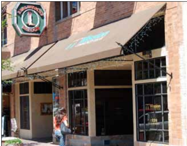
Awning with decorative supports and open end.
