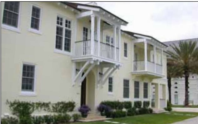
Minor differences in detailing and fenestration articulate the units.
