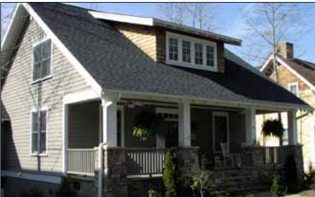
One-and-a-half story cottage house with integral porch.
