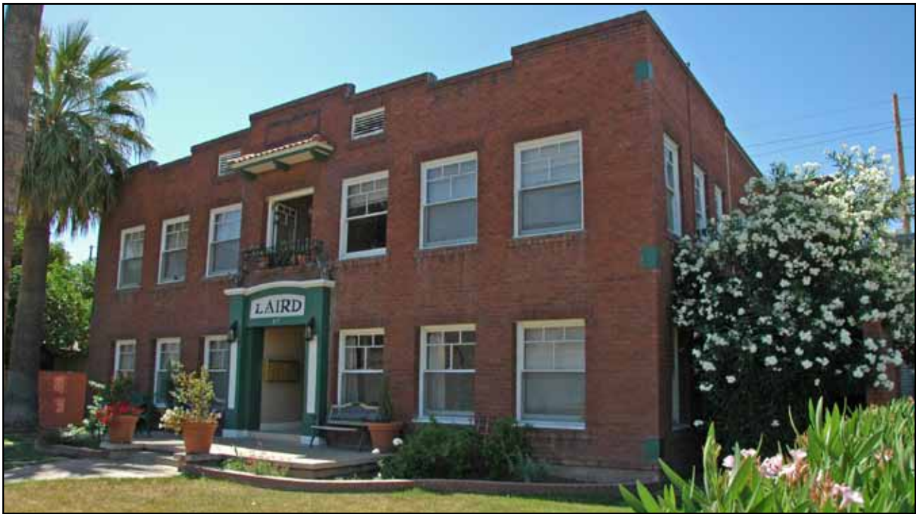
An apartment house with a recessed stoop.
