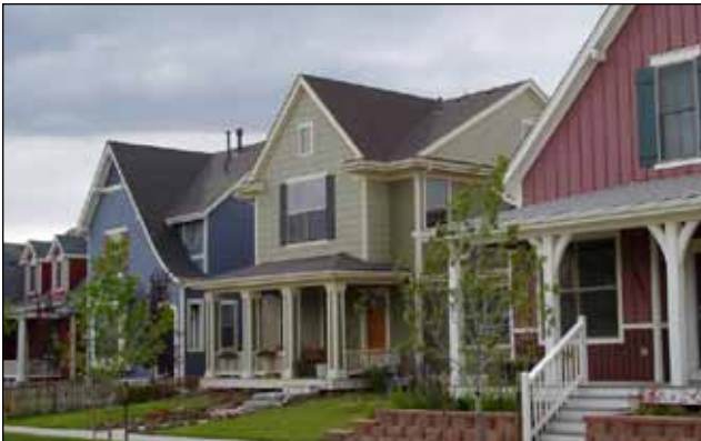
Newly constructed two-story cottage houses
