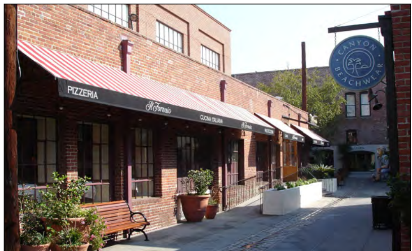
Series of awnings along a frontage.
