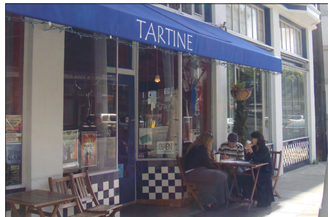
An example of a shopfront with a recessed doorway.
