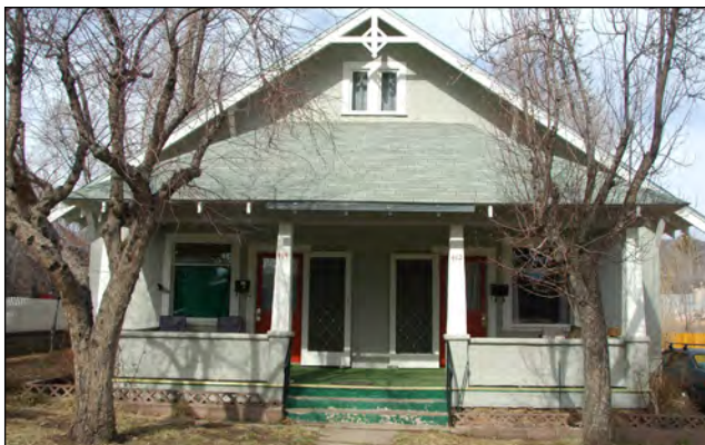
A side-by-side duplex with a shared porch.
