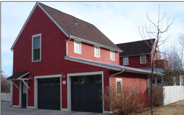
One-and-a-half-story carriage house with an internal stair.
