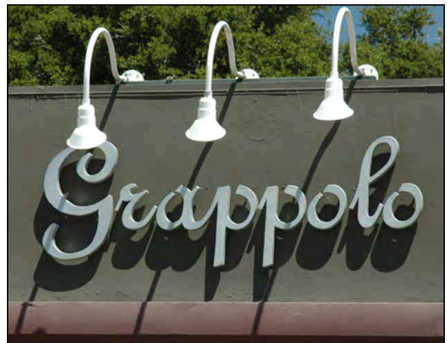
Metal wall sign, offset from building facade.
