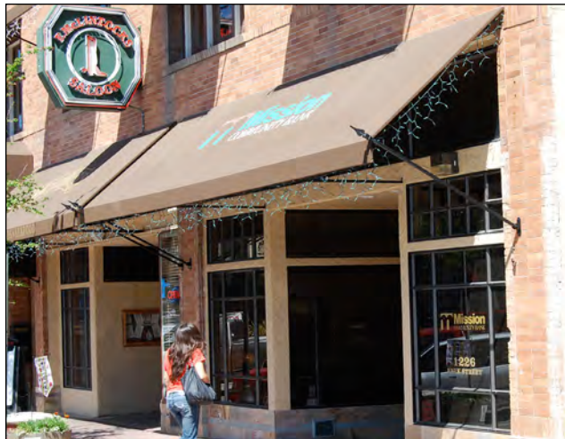
Awning with decorative supports and open end.
