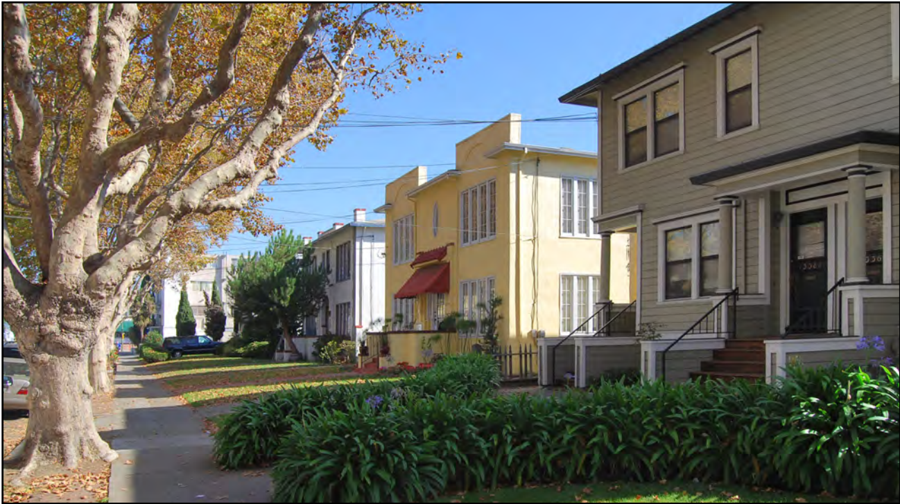
A group of apartment houses that have the scale and character of large single-family houses.
