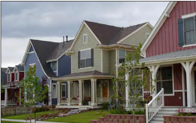
Newly constructed two-story cottage houses
