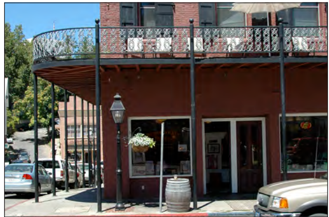
A one-story gallery with second floor access.
