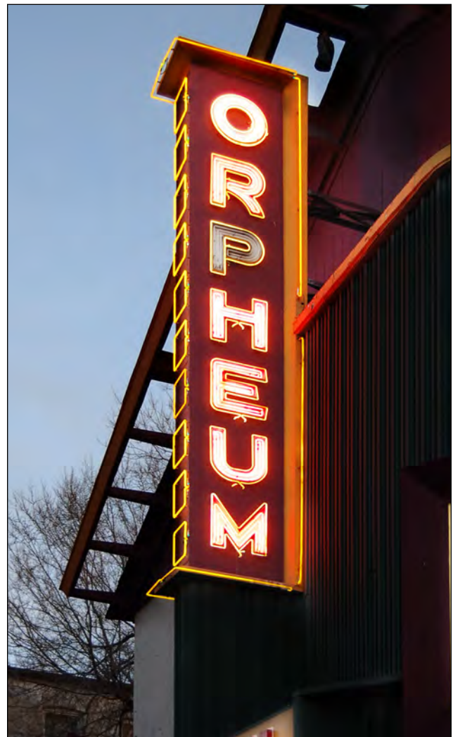
Lit marquee sign; neon lettering used in conjunction with painted lettering.
