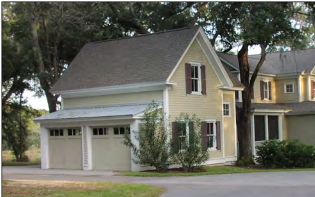
One-and-a-half-story carriage house.
