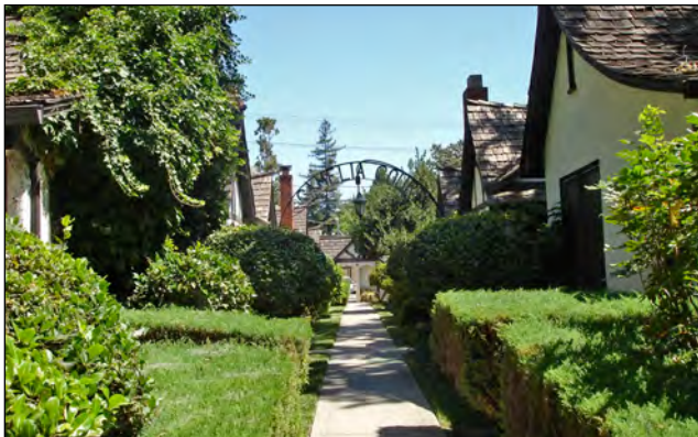
Bungalow court with a heavily landscaped court.
