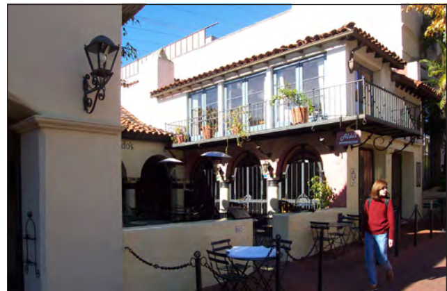
This commercial forecourt provides an outdoor dining area along a vibrant commercial street. The ROW is defined by a low wall as required by this Code.
