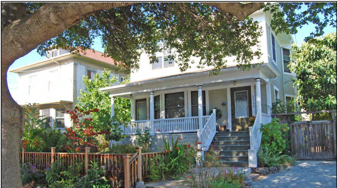
The difference in the form between this duplex and single-unit houses in the neighborhood is barely perceptible.
