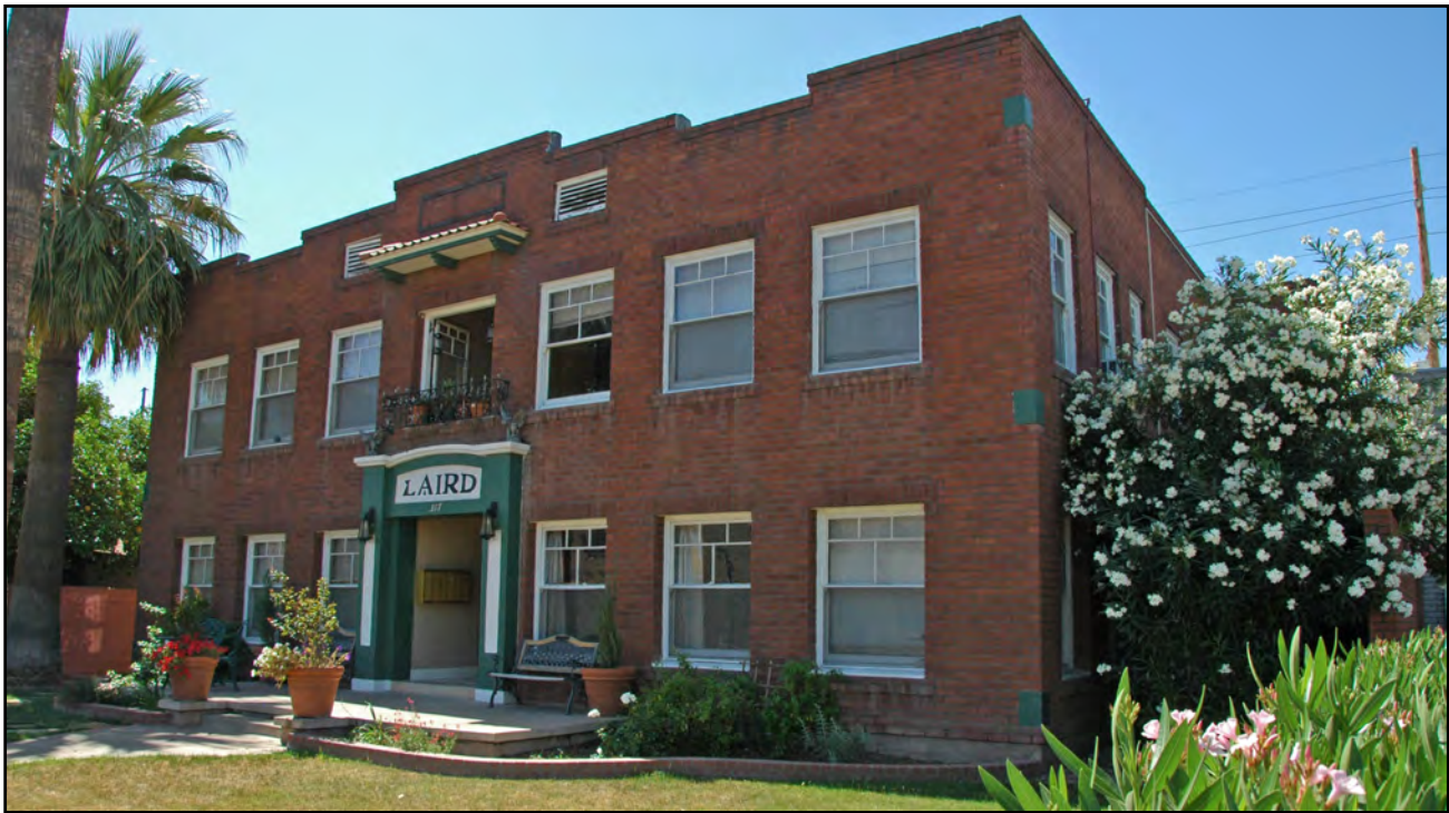
An apartment house with a recessed stoop.
