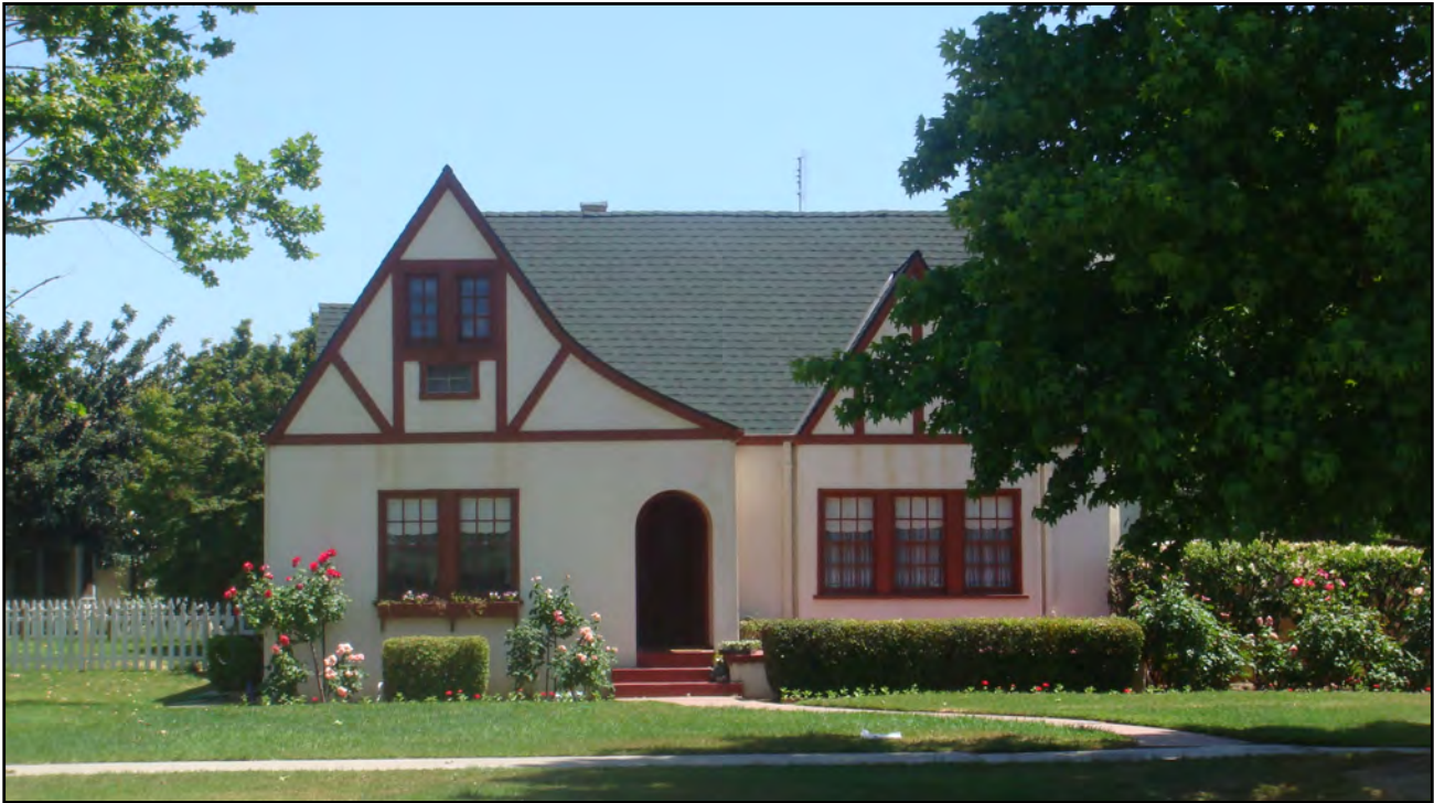
One-and-a-half-story front-loaded village house.
